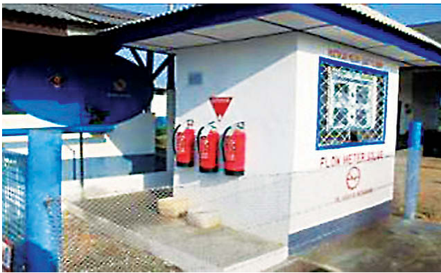
Safe storage of inflammable material
